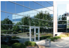
Diebold, Inc. Green Office Addition + Renovation
