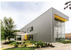
SoL Harris/Day Architecture New Corporate Office
