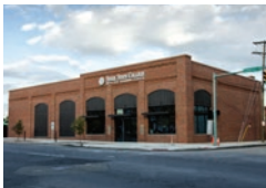
Wellsite Training Center Advanced Learning Center Renovations
