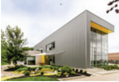
SoL Harris/Day Architecture New Corporate Office
