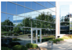
Diebold, Inc. Green Office Addition + Renovation
