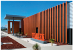
The Timken Company Mexico - New Plant + Offices
